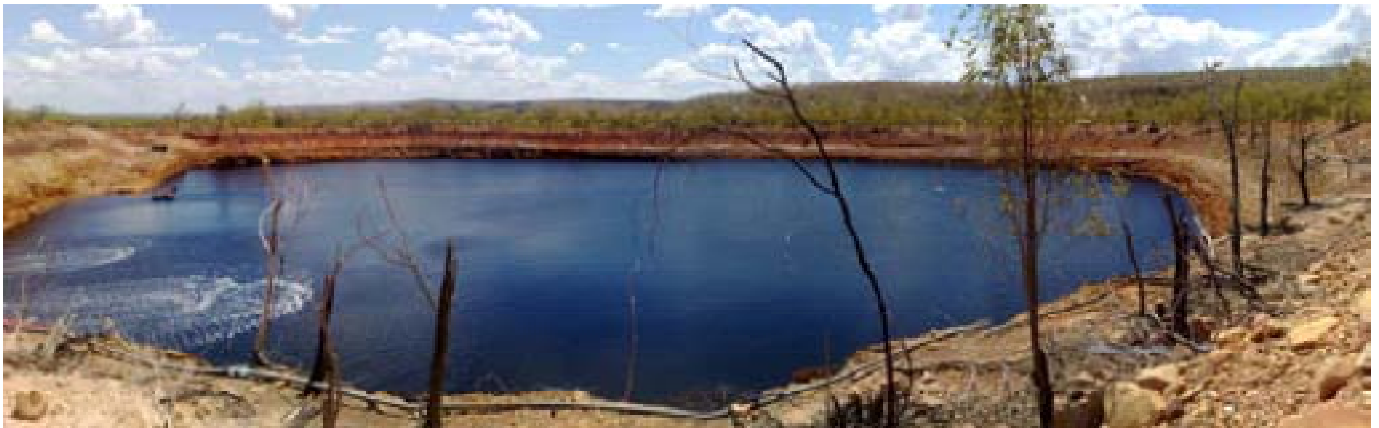
Sandy Flat Open pit looking north east – mined to a depth of 45 metres in mid 1990's
